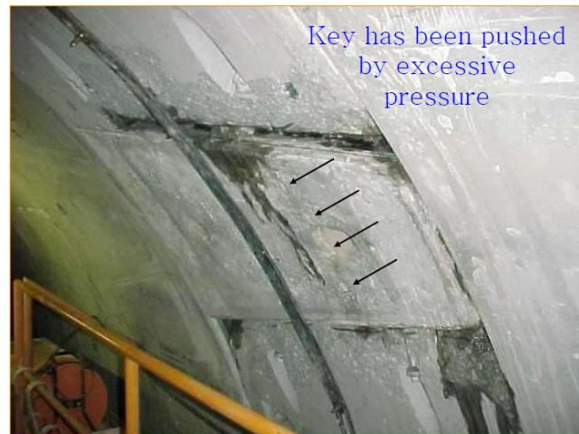
Figure 10 Key segment forced out of position (Dal Negro, 2006)
