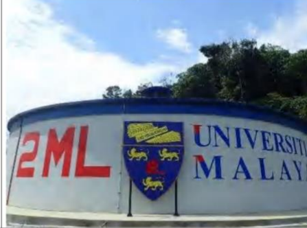
Tangki Simpanan Utama 2 (APM) Capacity: 2,000 m 3
