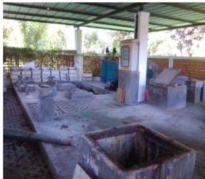
Example of Water Conservation - In Ground Water Tank (Institute Teknologi Sepuluh Nopember, Indonesia)
